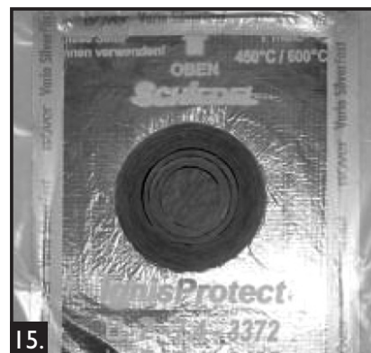
15. View of the finished vapour barrier sealed tightly all round.
