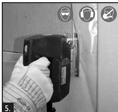
5. Make the opening. NOTE: Bearing elements must not be weakened! IMPORTANT: follow the safe working notes on page 29.
