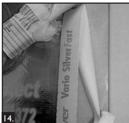
14. Secure the junctions with the vapour barrier by applying appropriate sealing tape to the foil lamination.
