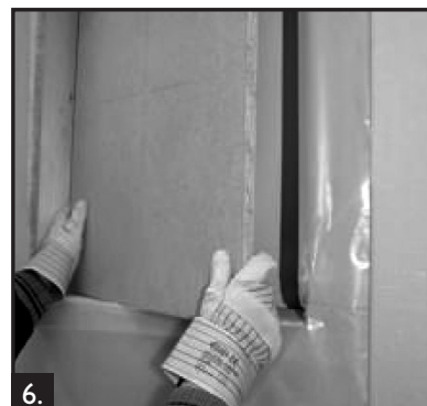
6. Remove wood fibre board, thermal insulation etc. from the assembly opening.
