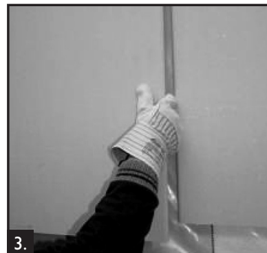
3. Remove plasterboard. NOTE: The vapour barrier must not be damaged!
