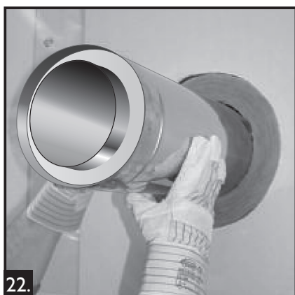
22. Example of a design with a double-walled connecting flue pipe.
