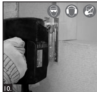
10. If necessary correct the opening. Replace the thermal insulation right around the assembly opening in the studwork. IMPORTANT: follow the safe working notes on page 29.
