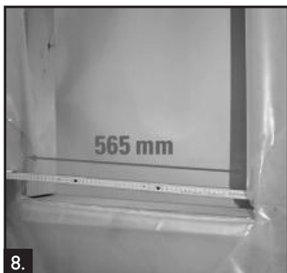
8. Check width of the opening: 565mm NOTE: Ignis-Protect must not be shortened on site!
