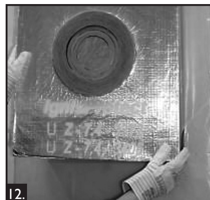
12. Insert Ignis-Protect so that it fits perfectly. The side laminated with foil should be facing inwards!
