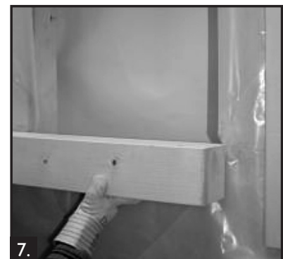
7. Install the wooden surround for Ignis-Protect into the studwork.
