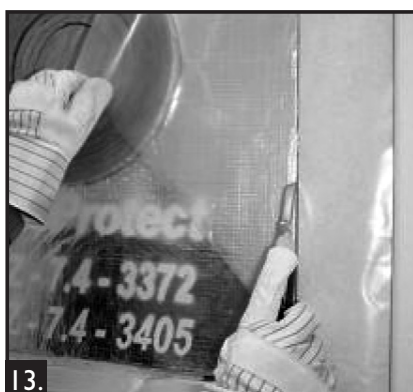
13. With Ignis-Protect in place, cut away the vapour barrier flush to the edges.
